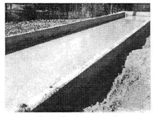
Fig. 1 - Fines decantation tank
